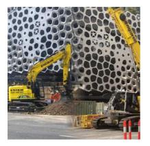
Preston Hire partnered with Geotech in getting piles in for the construction of the Brisbane Metro. A SY155U 16t limited swing excavator was used due to the restricted area of the jobsite.
